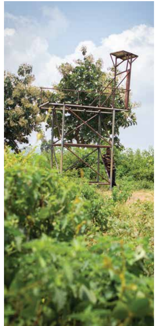
Abandoned water project in Kuzhako
