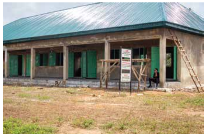
Newly constructed block of class room in Kuzhako (Primary School)
