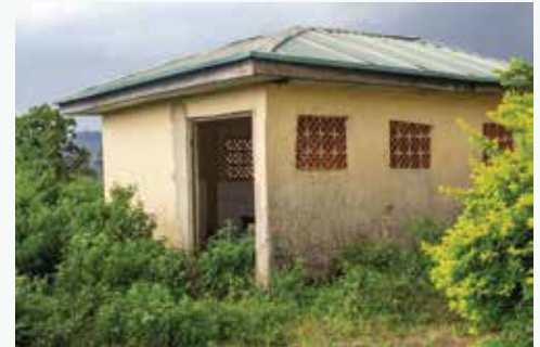
Abandoned Primary School Toilet in Kuzhako
